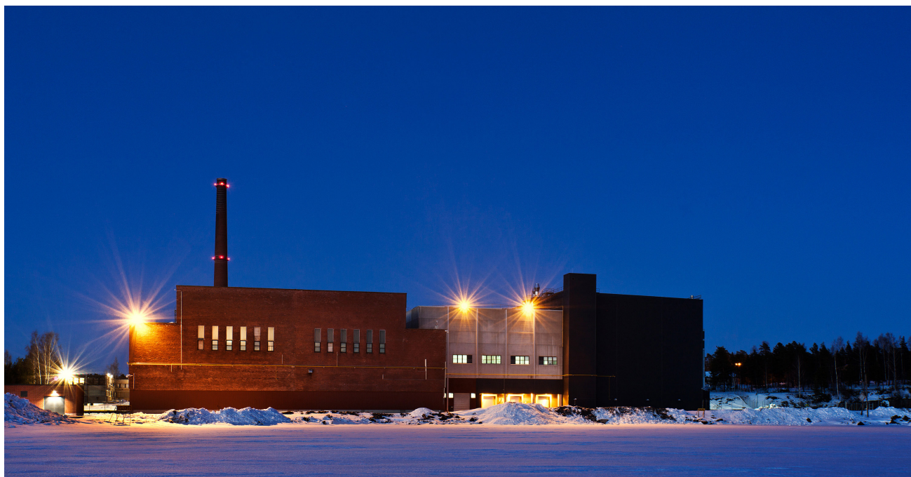
In Hamina, Finland, the recovered heat from Google's data centre is expected to cover approximately 80% of the annual heat needs for the Hamina district heating network, supplying about 2,000 households with sustainable heat free of charge.
