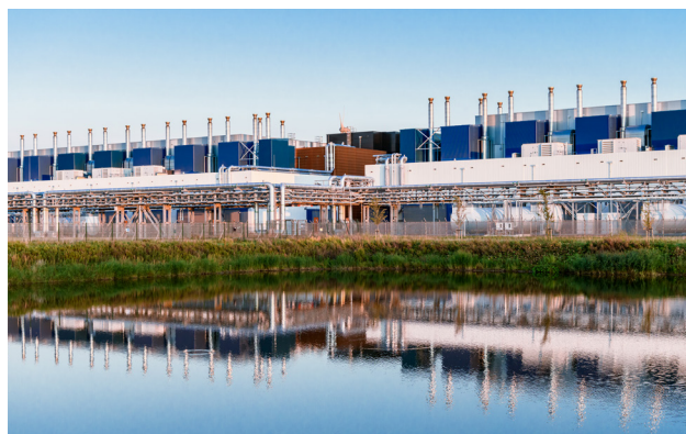
Clear waters reflect the beauty of our Eemshaven, Netherlands, data centre.
